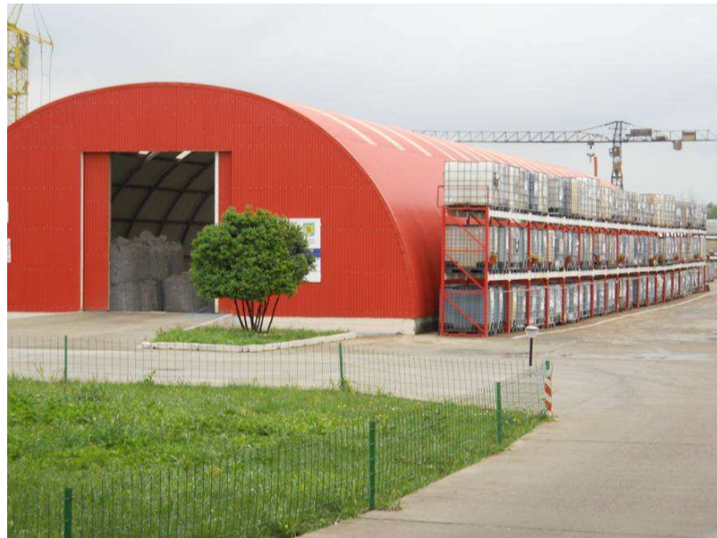
Figure 5: Set Car S. A. facilities in Braila
